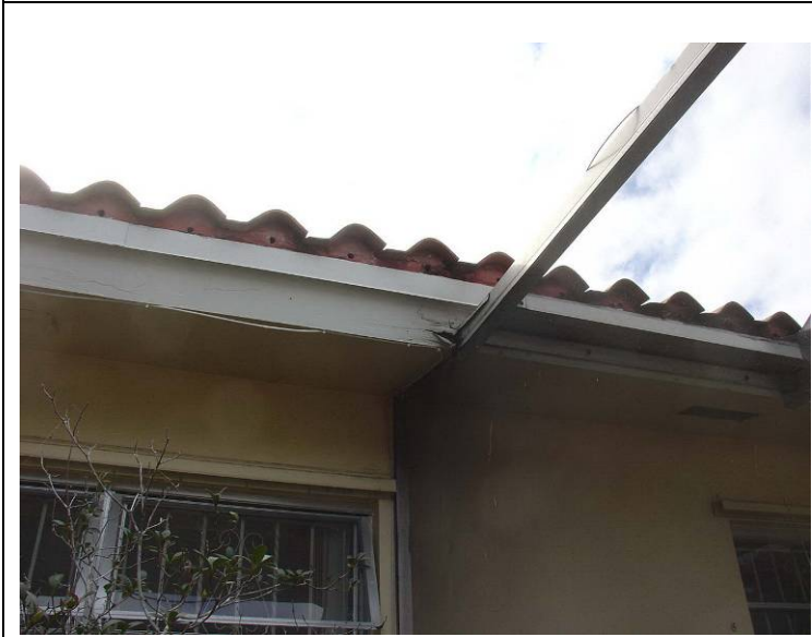
Damaged fascia and atrium screen enclosure.
