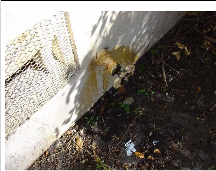
Main water supply shutoff valve.
